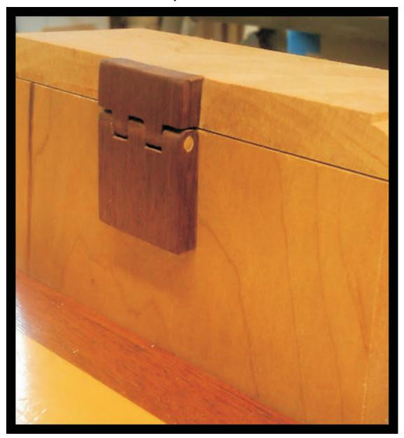
The glue is probably enough to hold the hinge in place but you could counter sink small brass screws for a better hold.
